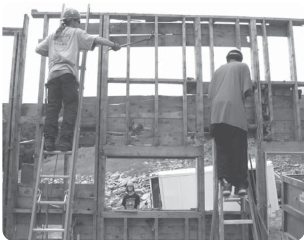
A YouthBuild crew deconstructs a building at Stowe Ski Resort.
